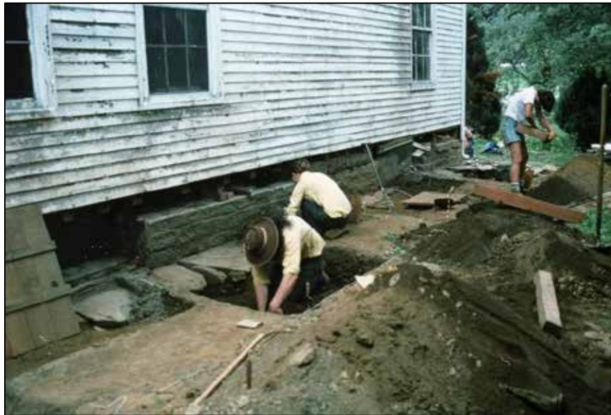
Figure 3: Archaeologists excavating around the foundation, ca. 1978. Note the large, flat “drip stones” along the exterior foundation wall.
