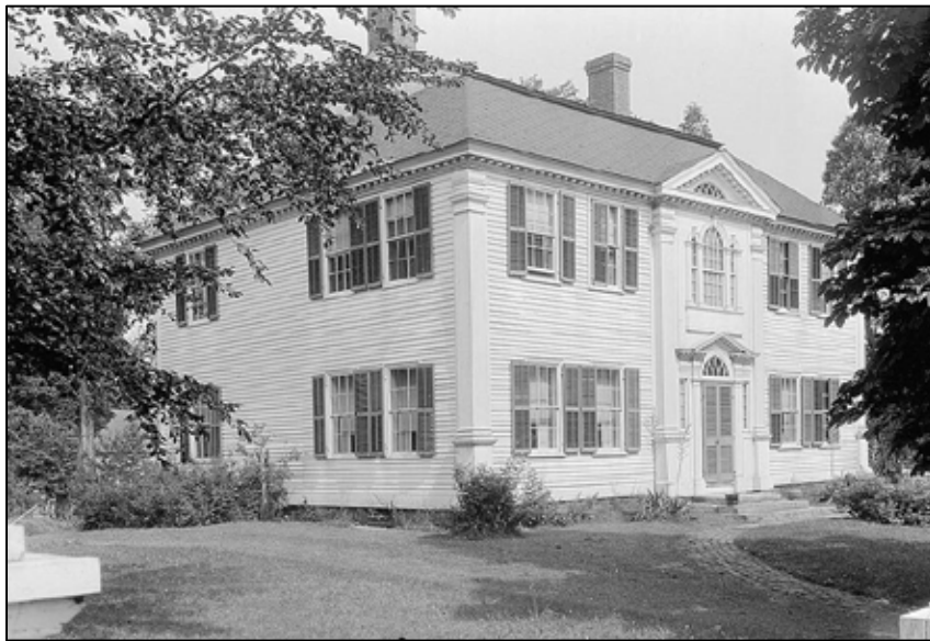
Figure 2. Photograph of the Luther Paine House, ca. 1940; Historic American Buildings Survey (HABS)
